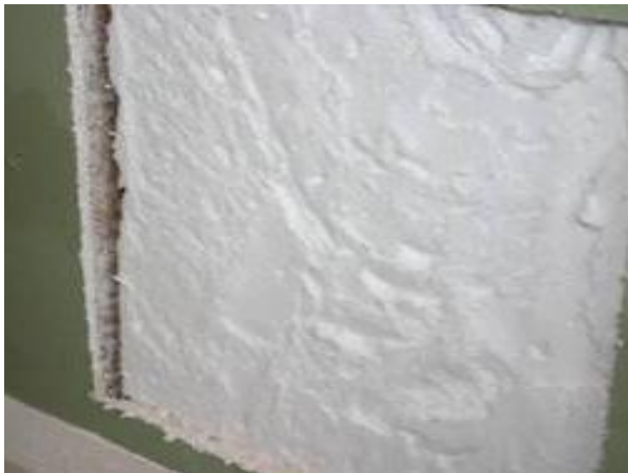
Figure 11: Removal of wallboard to assess Airfoam installation (House W3)
