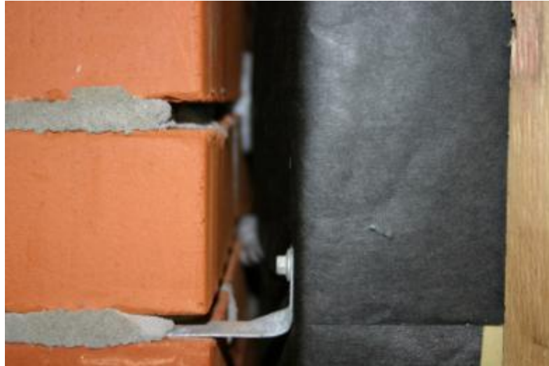
Figure 22: Cavity of Brick Veneer Wall (D4863a)
