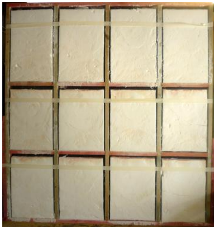
Figure 14: Test wall (D4861) after Airfoam installation and plasterboard removed
