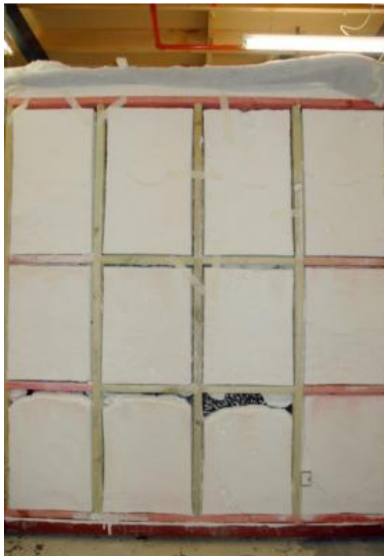
Figure 23: UFF-insulated brick veneer wall (D4863a) with plasterboard removed
